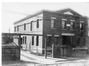
Former Waltham Water Works
