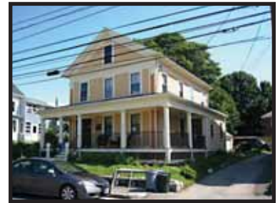
70 School St., Josiah Beard House, 1844, Greek Revival
